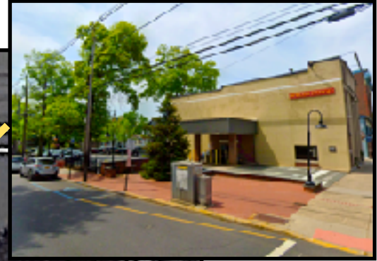
Side View from Bridge Street
