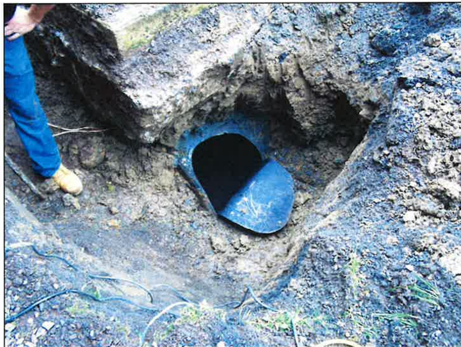
Photograph 4: View of the access hole cut into the side of the tank.
