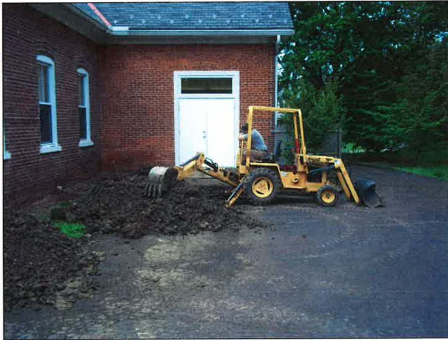
Photograph 1: Area where the UST was located.
