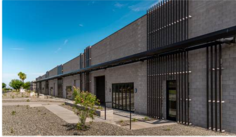
80x80 EXECUTIVE HANGAR EXTERIOR
