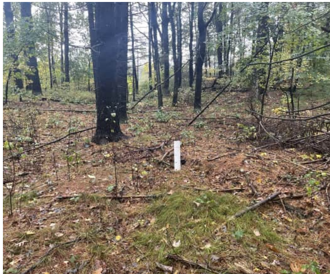
Photo shows typical 4-inch perforating PVC piping throughout the site.
