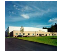
Keebler 17 Forge Park Franklin, MA 84,000 SF Completed in 1991
