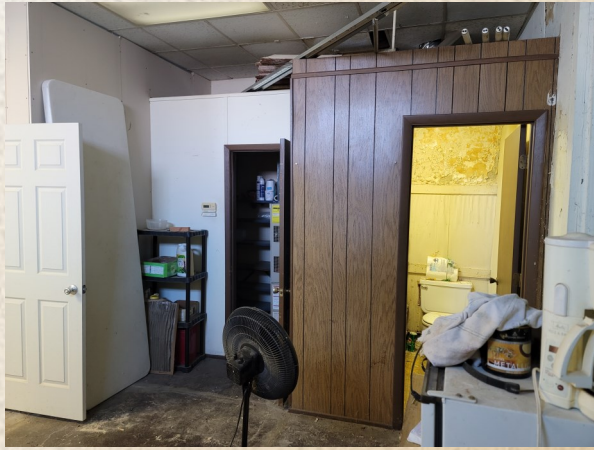
Street Front Building
