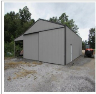
New Post Frame Utility Barn
