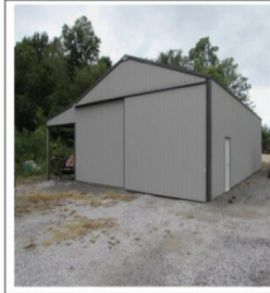
New Post Frame Utility Barn
