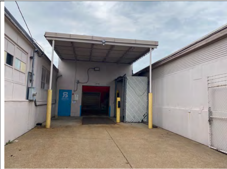
Entry into building
