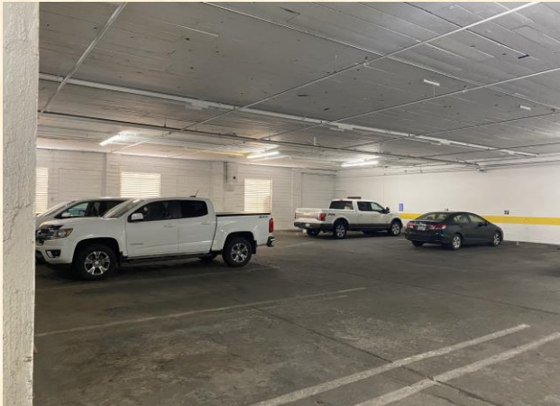
INDOOR PARKING GARAGE
