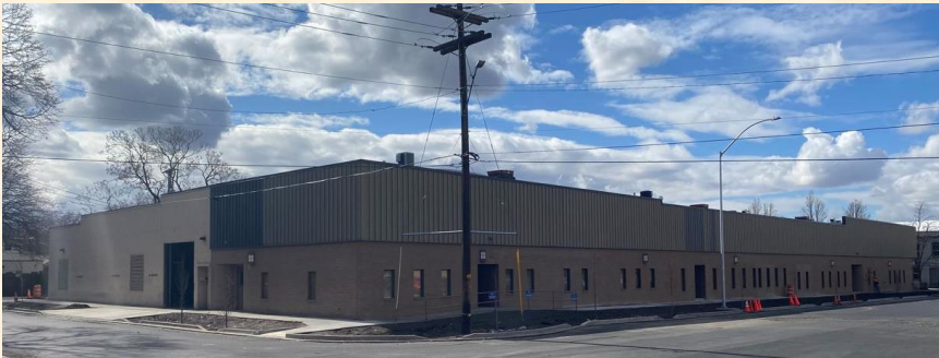
SECONDARY VIEW - E POPLAR STREET AT S COLVILLE STREET, WITH GARAGE ENTRY
