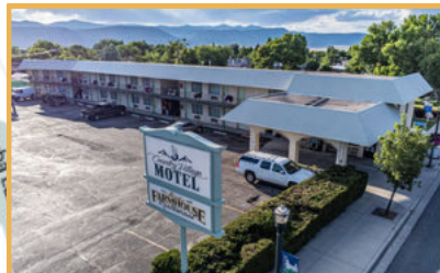
145 N MAIN STREET SUBJECT PROPERTY
