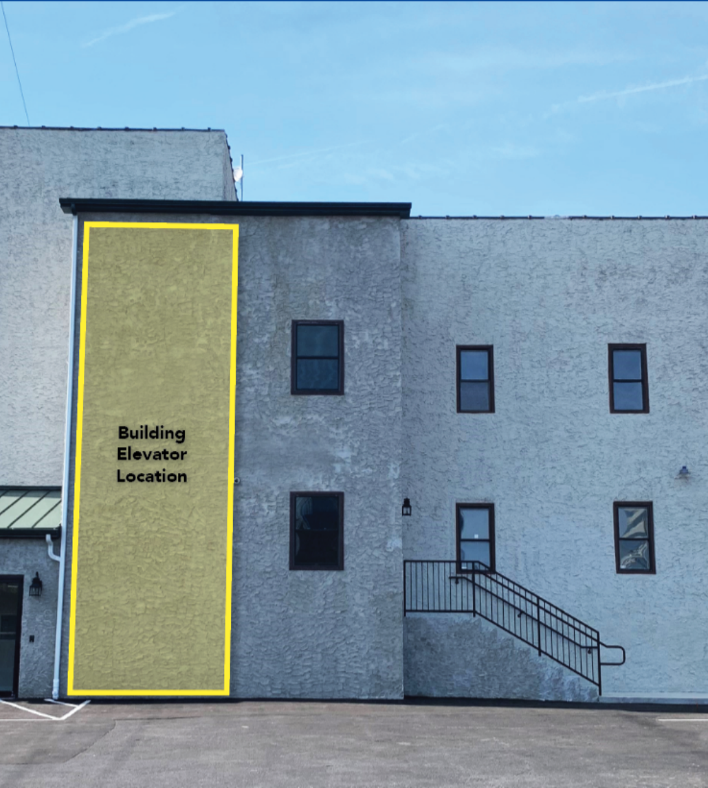
Exterior - Elevator Location
