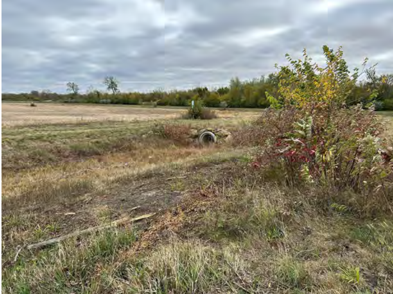
8. Drainage ditch and culvert along eastern boundary of Unit 3.
