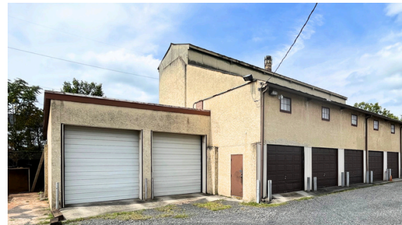
Second Floor of Main Storage Building with Mezzanine Space
