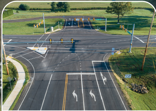
Connector Road Improvements - Completed 7/2022
