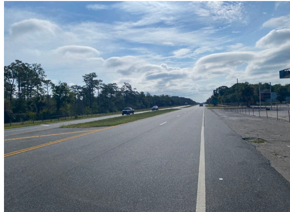
Looking West on State Road 16 Subject on Right Photo taken June 11, 2024
