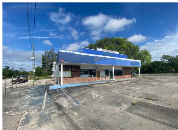
Front View of Convenience Store Photo taken June 11, 2024
