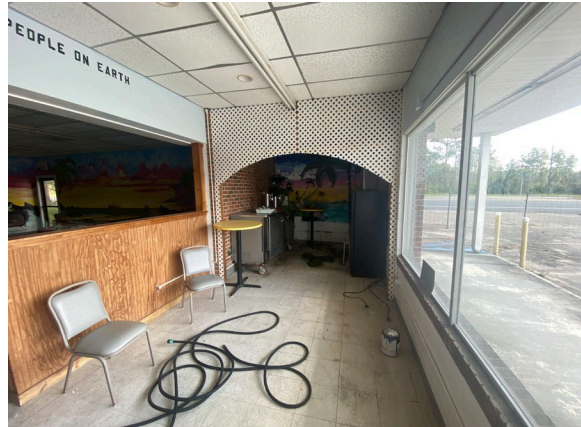
Interior of Restaurant Unit (Parcel One) Subject on Left Photo taken June 11, 2024
