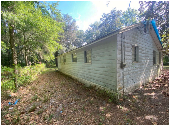
Westside View of SFR (Parcel Two) Photo taken June 11, 2024
