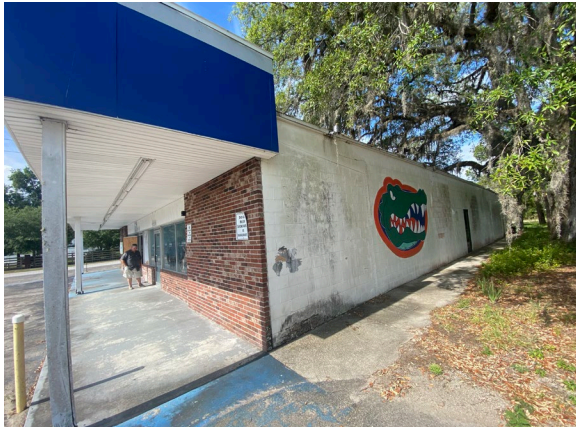
Northside View of Convenience Store (Parcel One) Photo taken June 11, 2024
