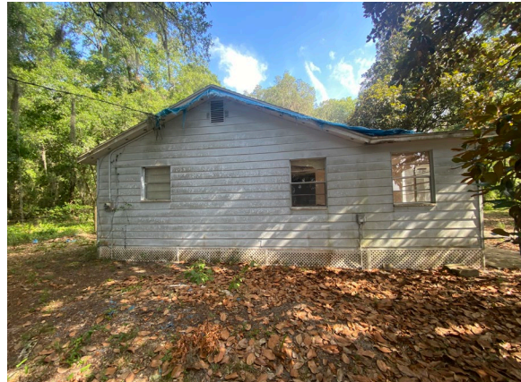
Front View of SFR (Parcel Two) Photo taken June 11, 2024
