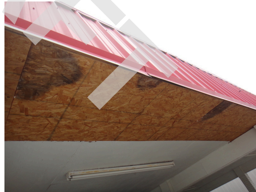
Damaged soffits
