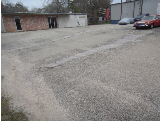
Fair asphalt paving
