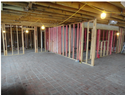
Interior overview bldg 1
