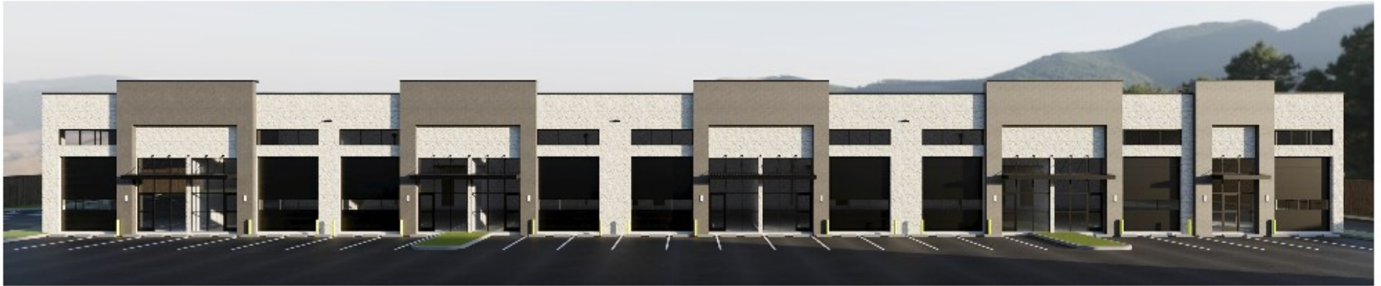
FLEX BUILDING FRONT VIEW
