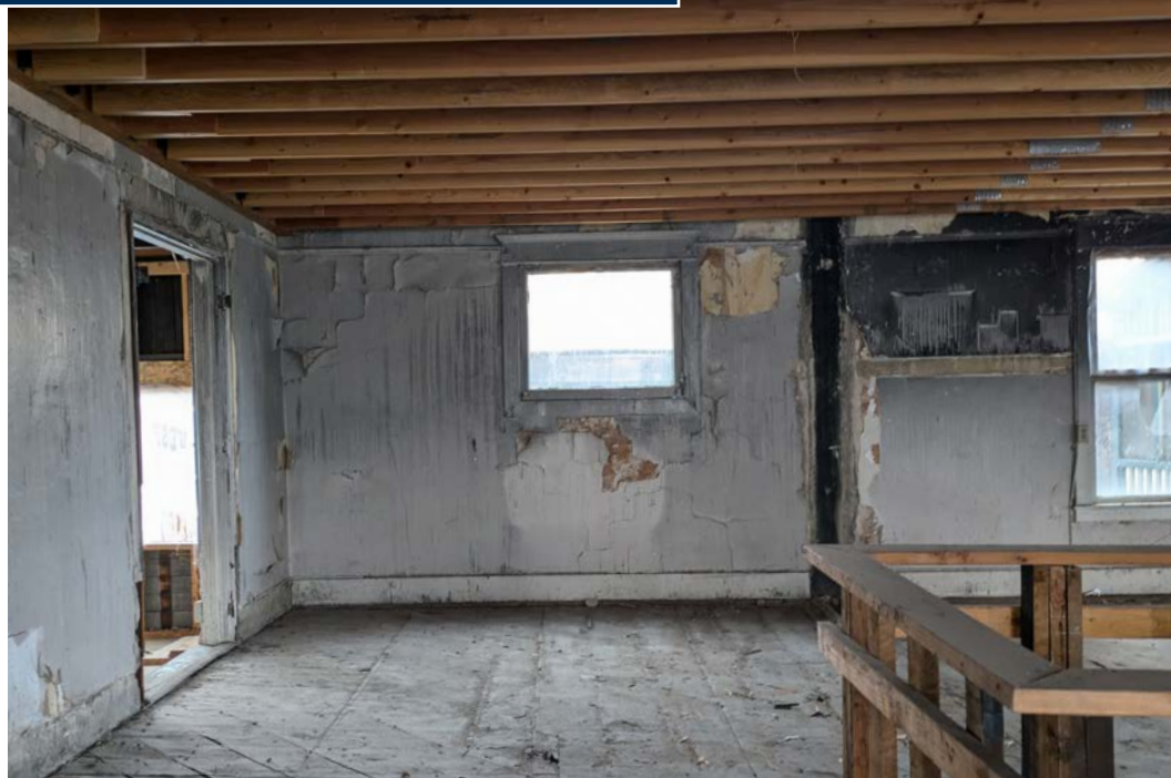
SHELL CONDITION WITH NEW ROOFING & TRUSSES
