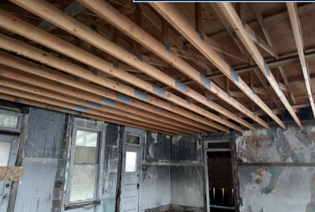
SHELL CONDITION WITH NEW ROOFING & TRUSSES
