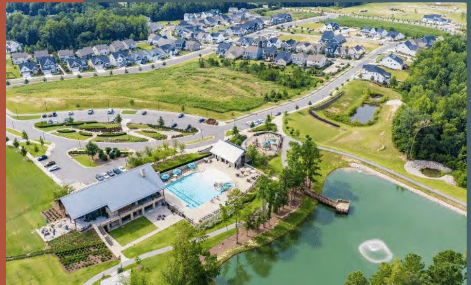
Wendell Falls, one of Wake County's largest mixed-use master-planned communities
