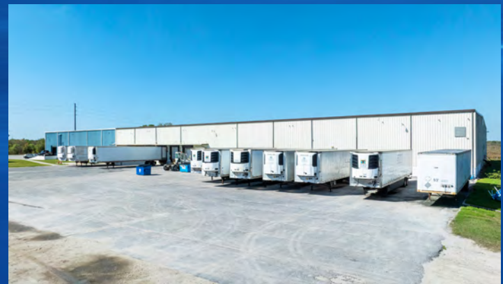
WAREHOUSE LOADING DOCKS
