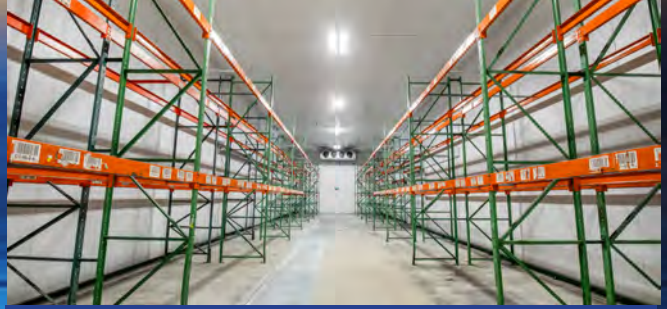
WAREHOUSE FREEZER AREA
