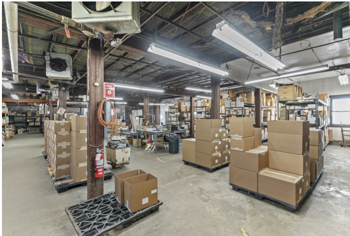
Single Story Warehouse
