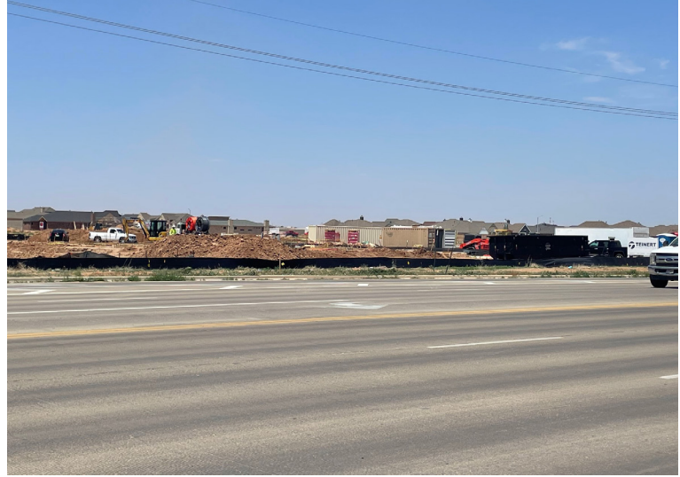
MCDONALD'S AND ALLIANCE CREDIT UNION UNDER CONSTRUCTION
