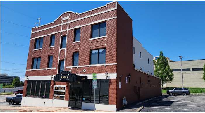
BUILDING FRONT, NORTH PARKING
