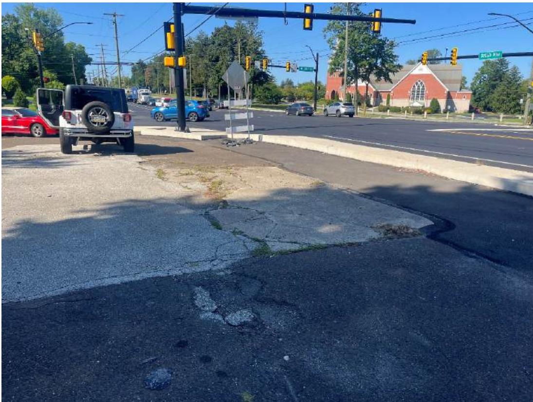
Photo 4 – Former dispenser island location
