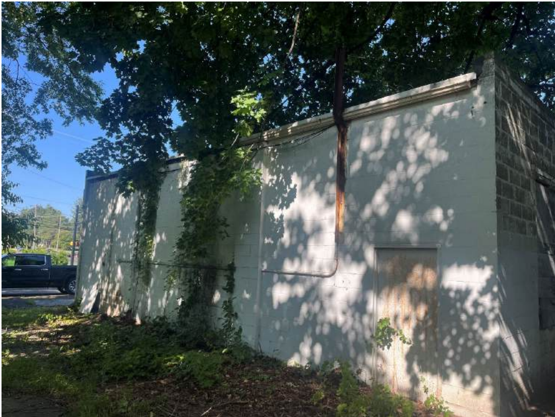
Photo 8 – View of the rear of the building
