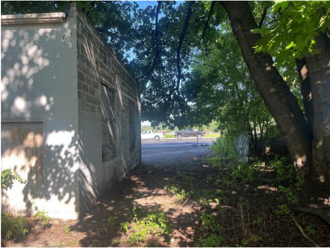
Photo 5 – Northern building elevation
