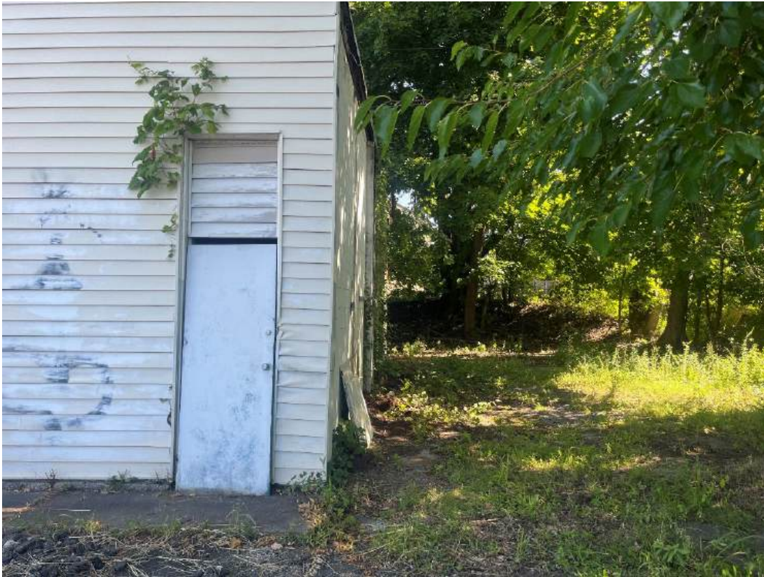
Photo 3 – Overgrown area to the east of the building
