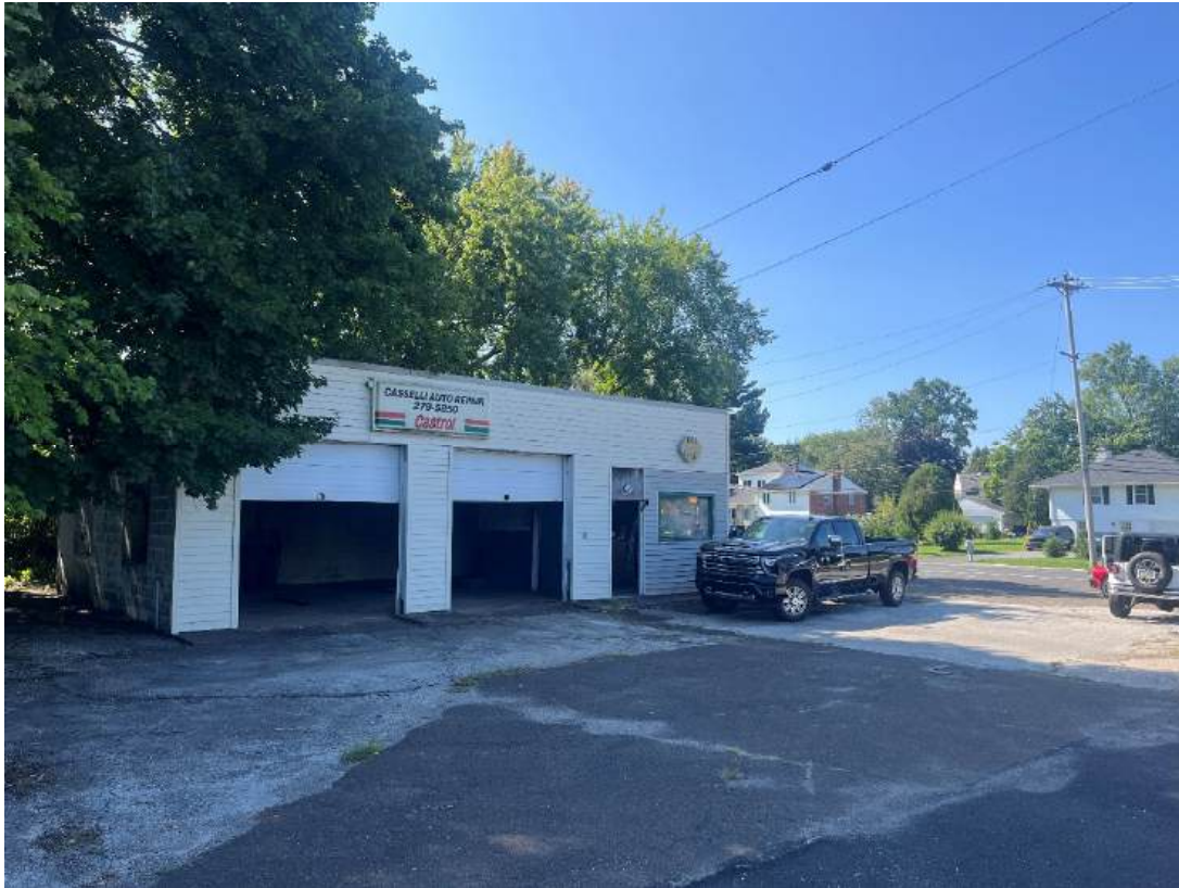
Photo 1 – View of Subject Property from Dekalb Pike
