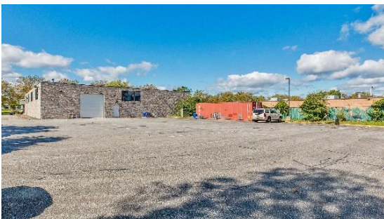
Oversized Large Yard
