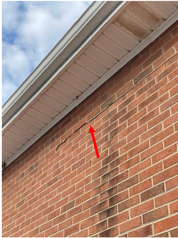
Parapet shift on east wall
