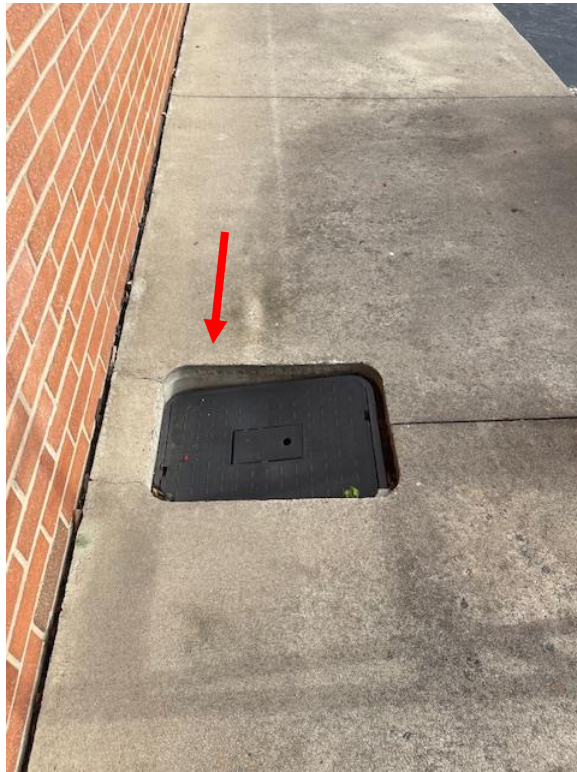
Water meter settlement on east wall
