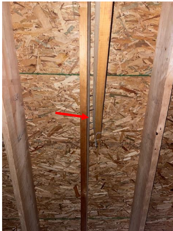
Collar ties with nail failure
