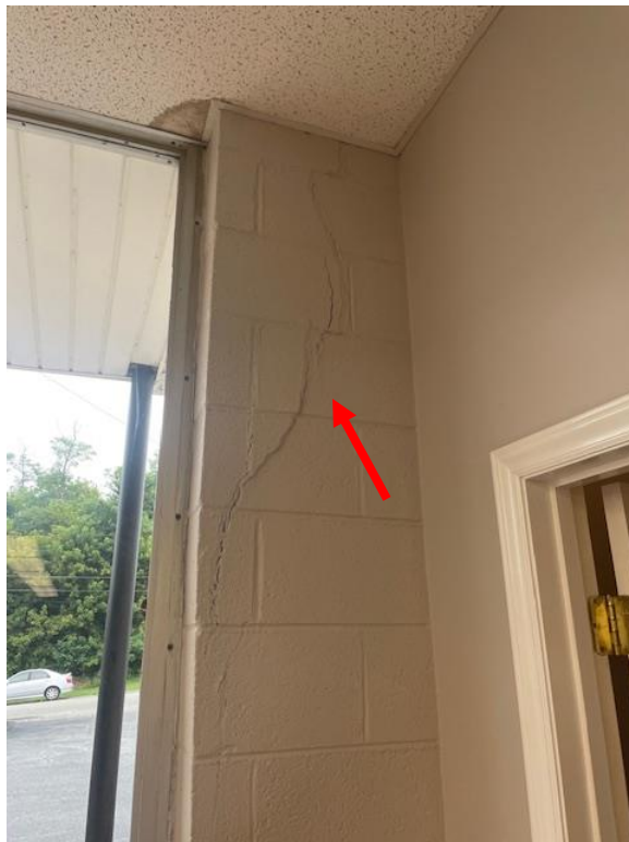
Wall settlement crack on north wall
