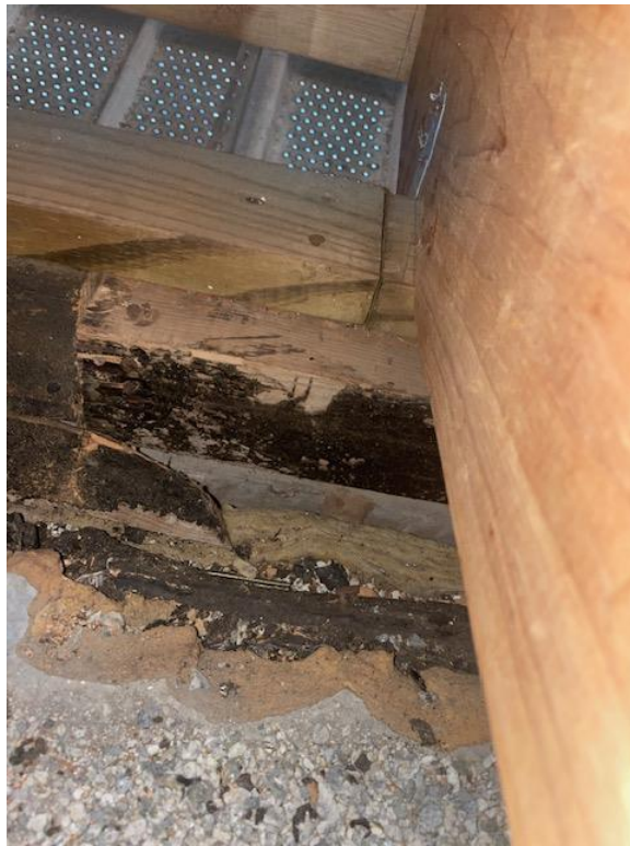
Pushed out rafter bearing plate on east wall
