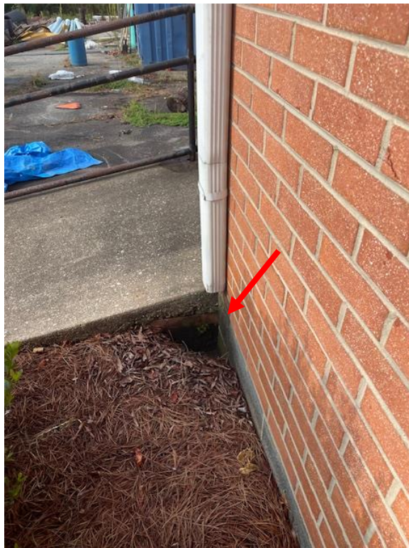
Downspout discharge issue on east wall – trip hazard
