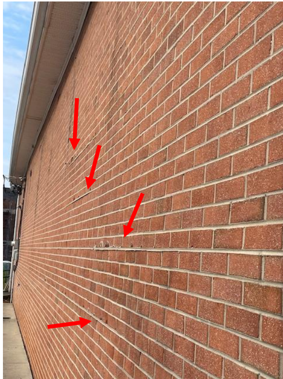
Joint spauling on east wall
