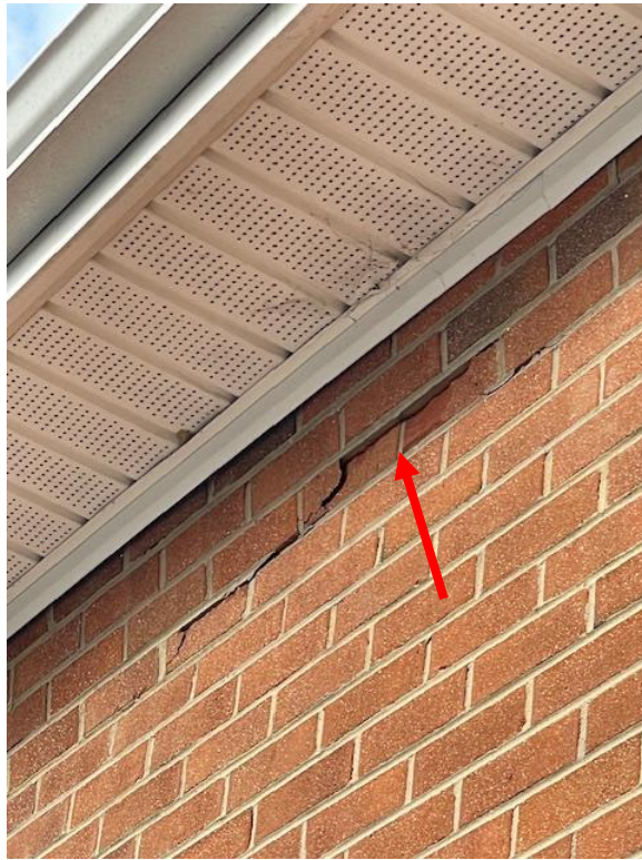
Parapet shift on east wall
