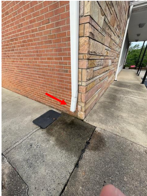
Downspout discharge issue on east wall
