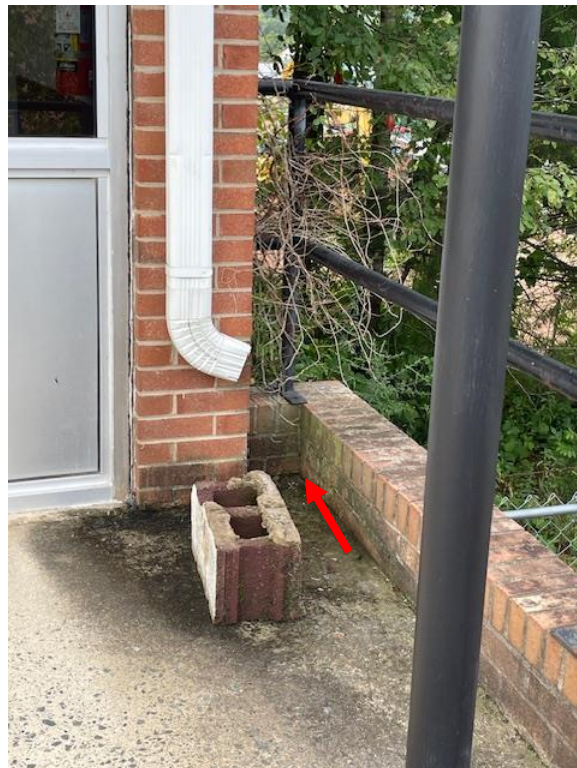
Downspout discharge issue on west wall
