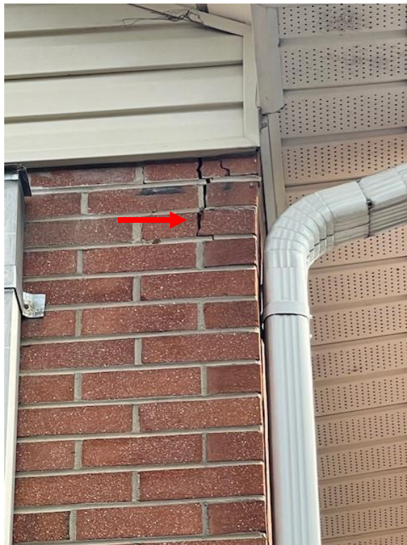
Parapet shift on east wall
