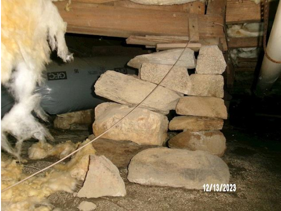
STRUCTURAL FRAME AND BUILDING ENVELOPE: typical stacked stone pier
