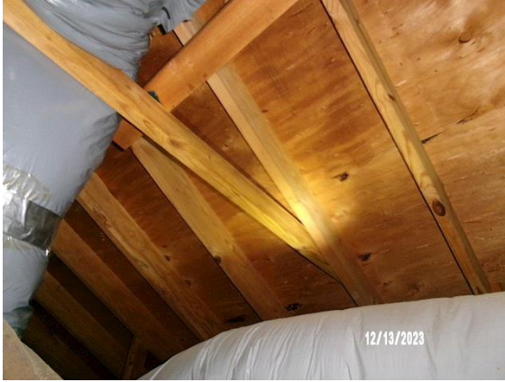
Attic / Roof Framing and Sheathing: framing visible above drop ceiling
