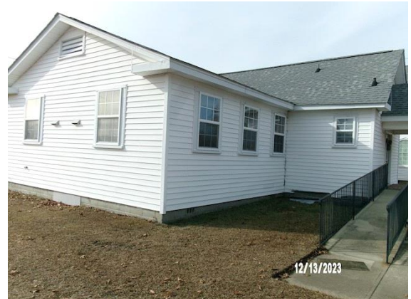
GRADING / DRAINAGE: typical near level to level grade along foundation
