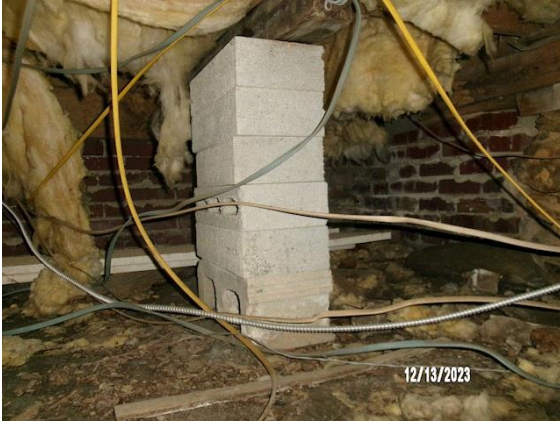
STRUCTURAL FRAME AND BUILDING ENVELOPE: typical dry-stacked block pier
