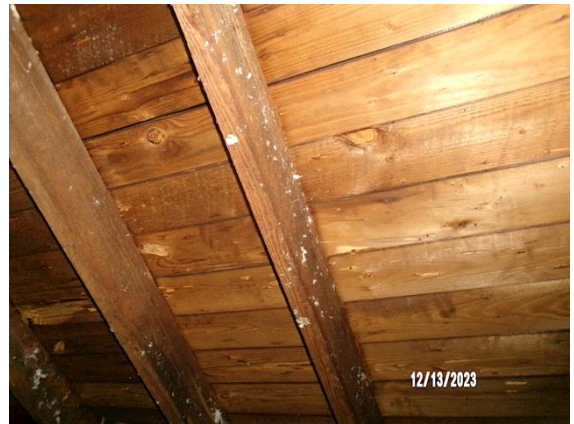
Attic / Roof Framing and Sheathing: framing visible from ceiling scuttle
