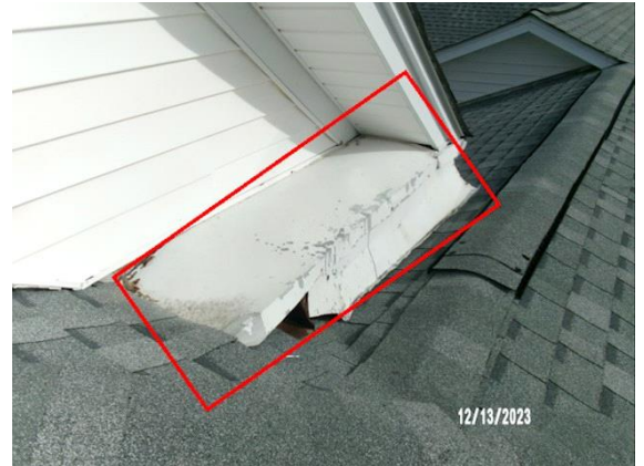
EXTERIOR SURFACE: back left water table / return
