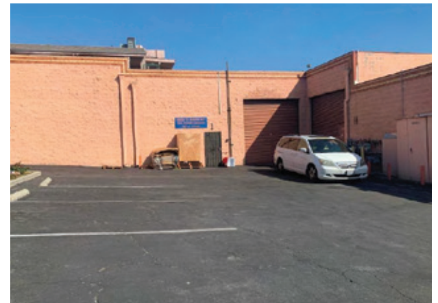
COMMERCIAL KITCHEN UNIT
