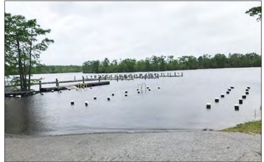
Town Docks. This shows a view of the boat launch area looking toward the docks. This was taken after a rain event, not a storm, so it's clear from this picture that the docks and piers need to be replaced with floating docks.
