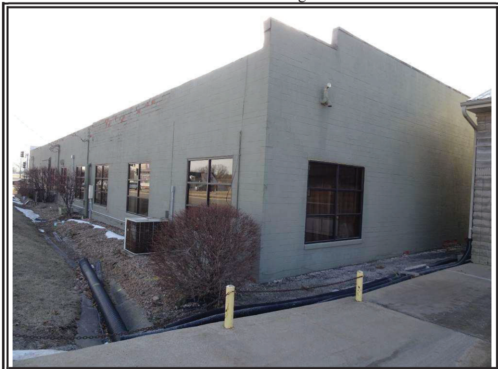
Rear of Building
