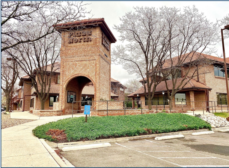
Plaza North Entrance
