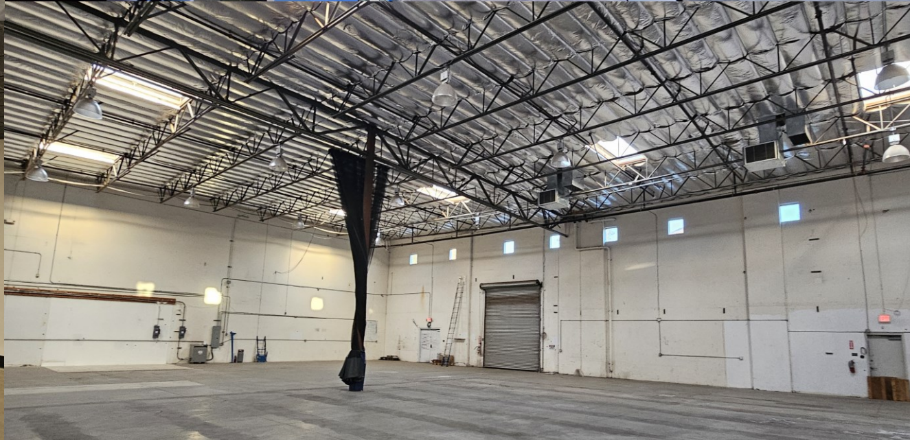
Natural Light in 24' Warehouse, 1200 AMP
