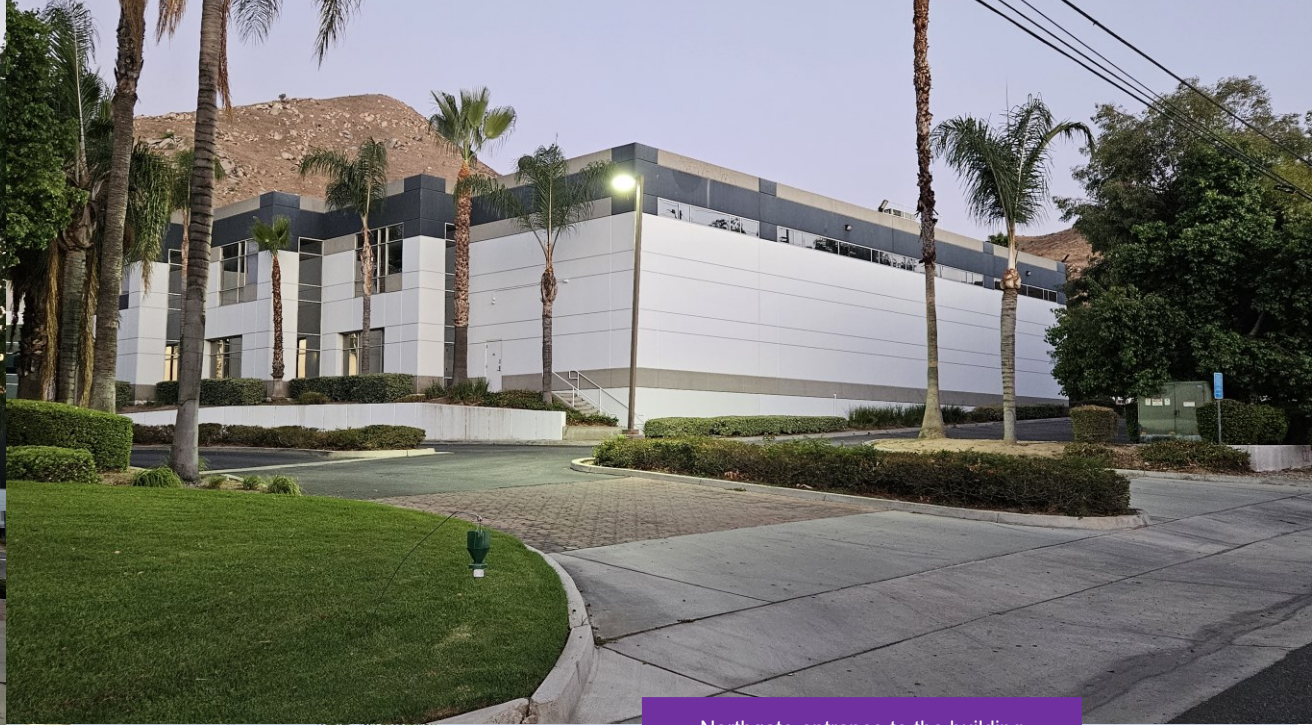
Northgate entrance to the building
