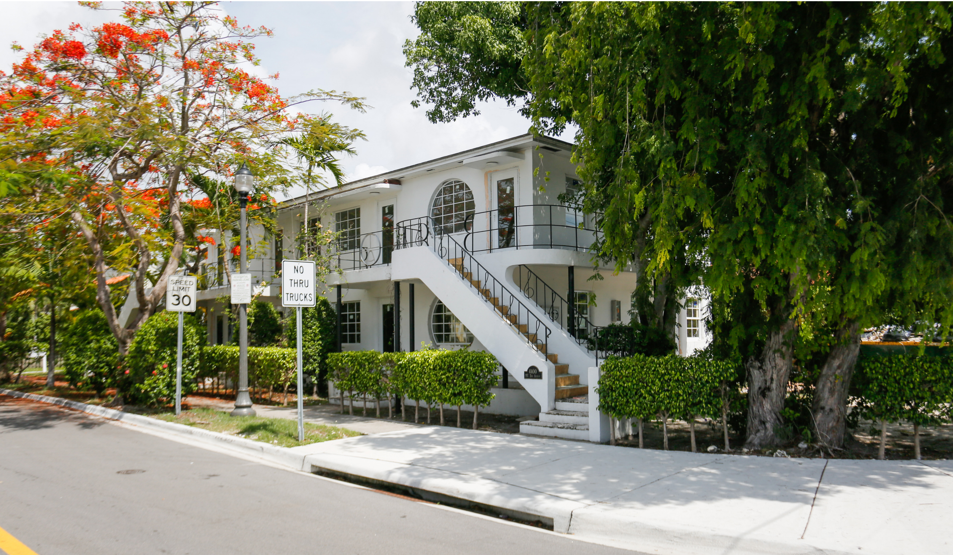
EXISTING - BUILDING PHOTOS
