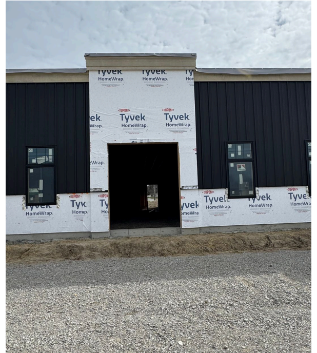
Current Construction (March 2026)
