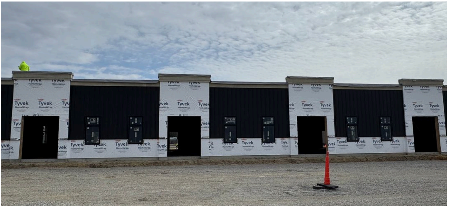
Current Construction (March 2026)
