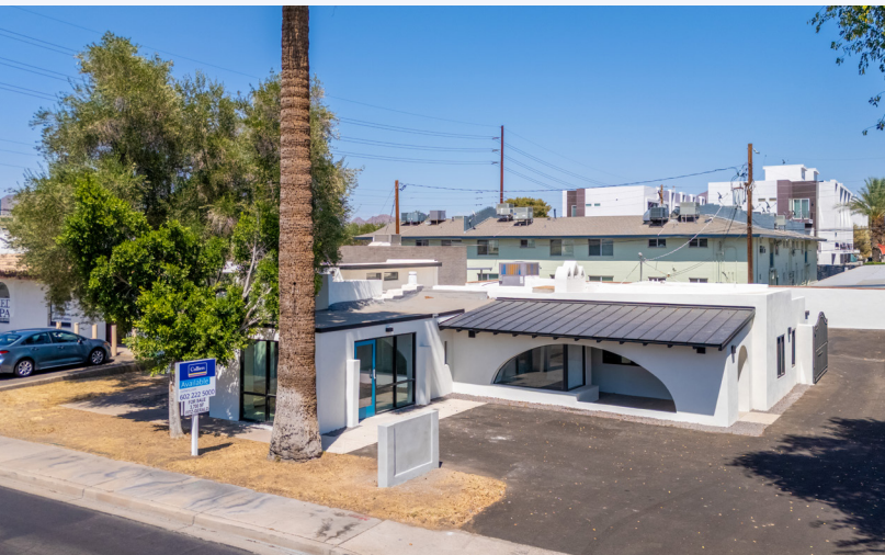
Live look at renovation set to be completed August 1, 2026
