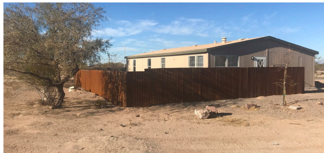
STEEL ENCLOSED BACKYARDS
