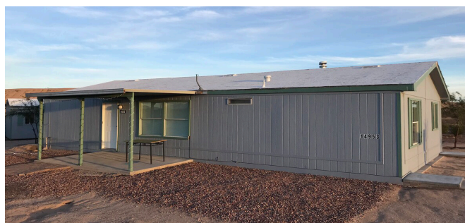
UPGRADED WINDOW COVERINGS
