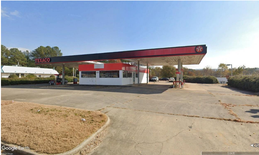
Figure 1 View of the existing site.
