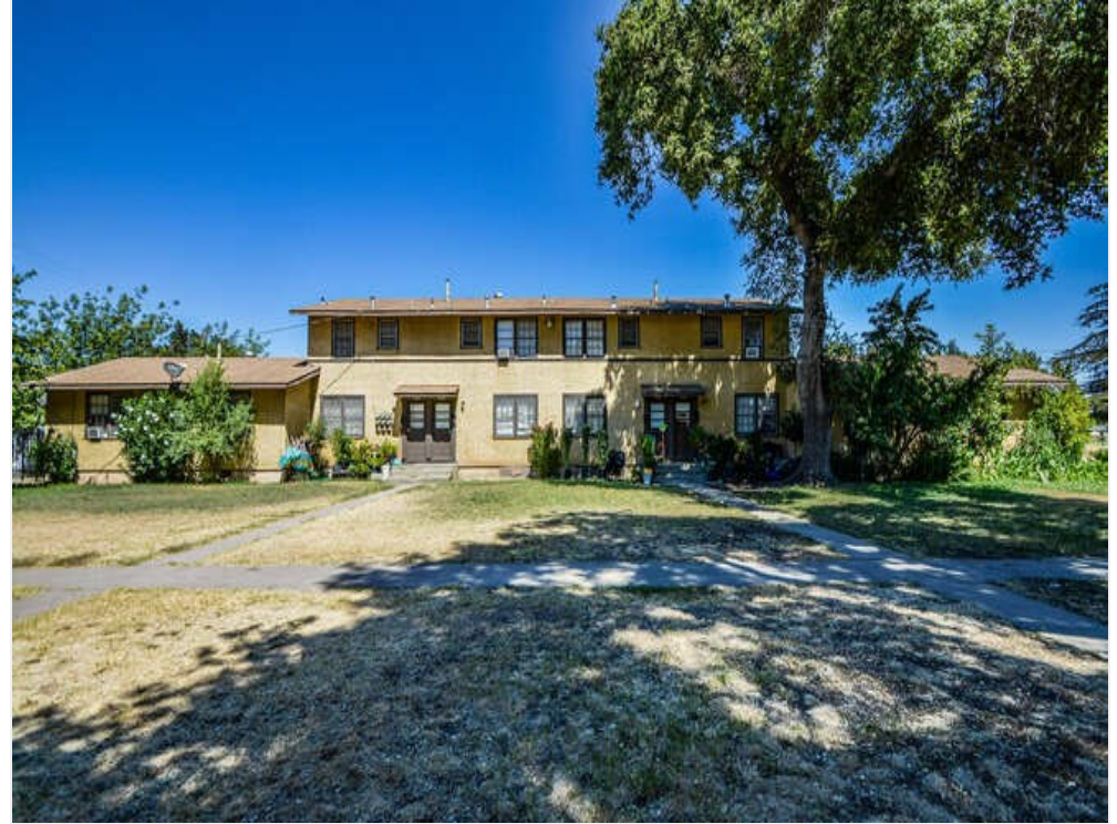
1572 and 16081614 E 6th St-small-020-017-Front of Building 3 for 1572 E-666x417-72dpi
