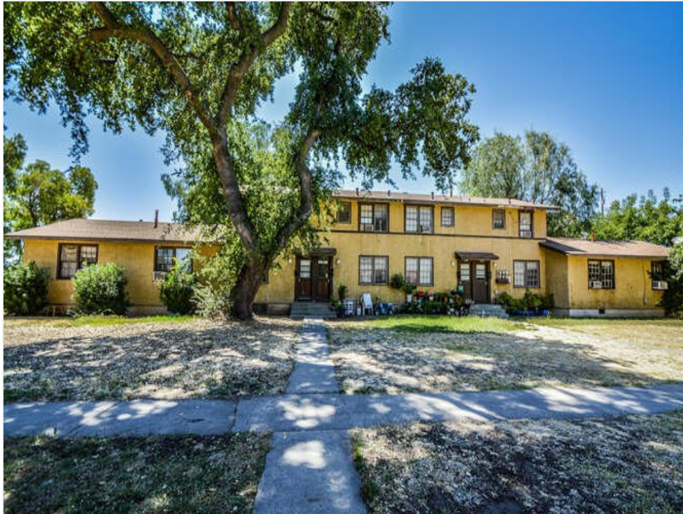
1572 and 16081614 E 6th St-small-018-023-Front of Building 1 for 1572 E-666x417-72dpi
