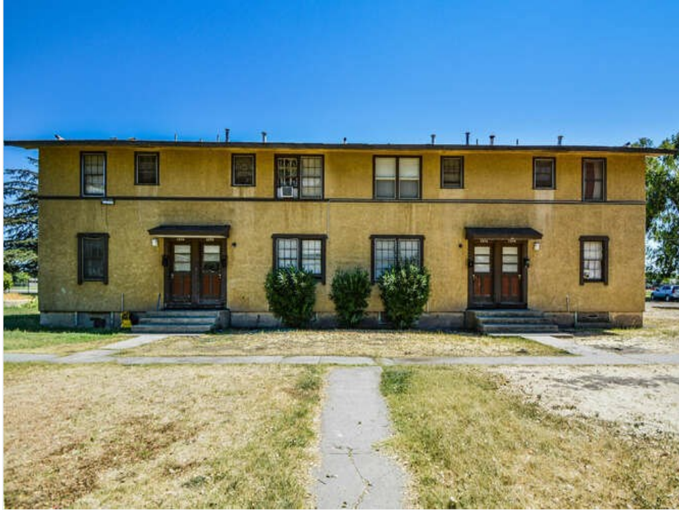
1572 and 16081614 E 6th St-small-019-015-Front of Building 2 for 1572 E-666x446-72dpi
