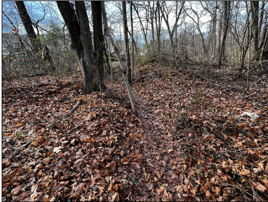
Photo 4: View of offsite drainage swale from King Phillips Drive, looking west.
