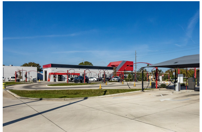
Covered vacuum canopy, tunnel entry and queuing lanes
