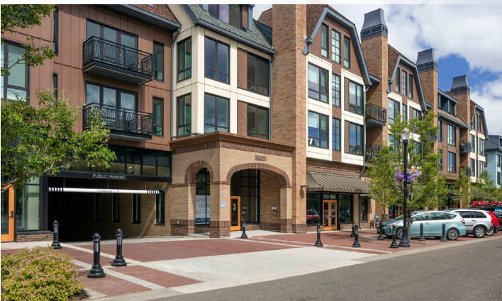
VIEW OF GARAGE INGRESS/EGRESS OFF FIRST STREET & ADJACENT PEDESTRIAN INGRESS/EGRESS
