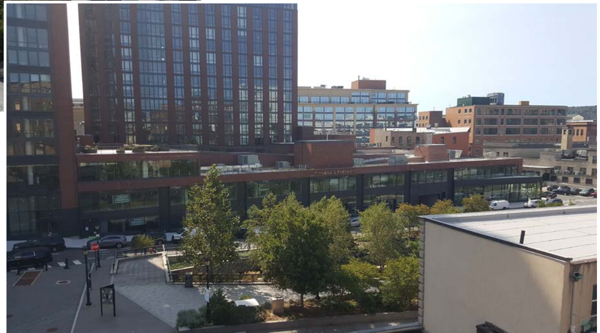
ROOF VIEW FACING SAWYER PLACE & AREA RETAIL
