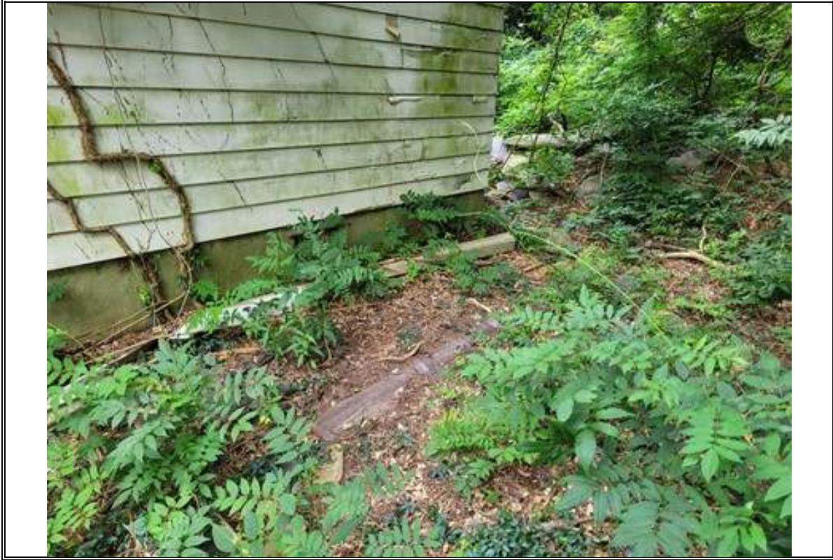
Photograph Number 1: View of metal structure
