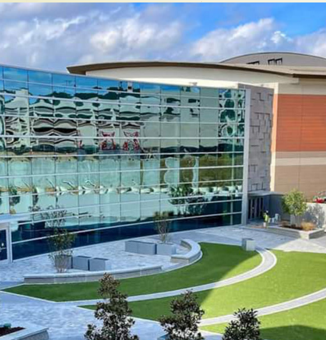
GAS SOUTH CONVENTION CENTER
