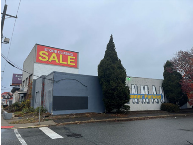
Exterior View of the Subject.
