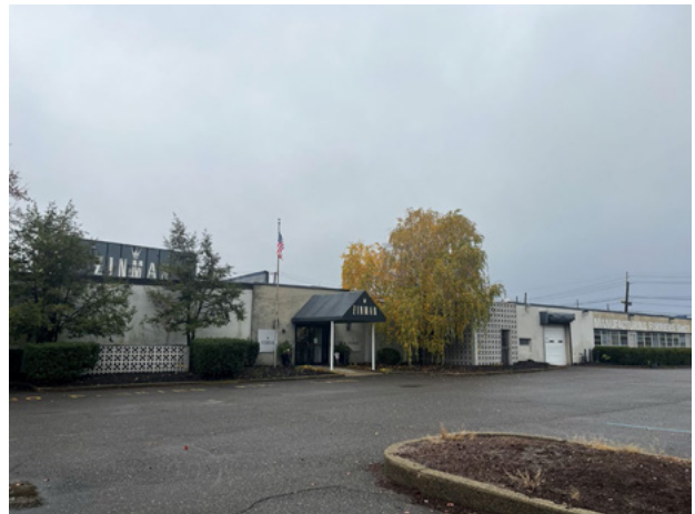
View of the Main Entrance.
