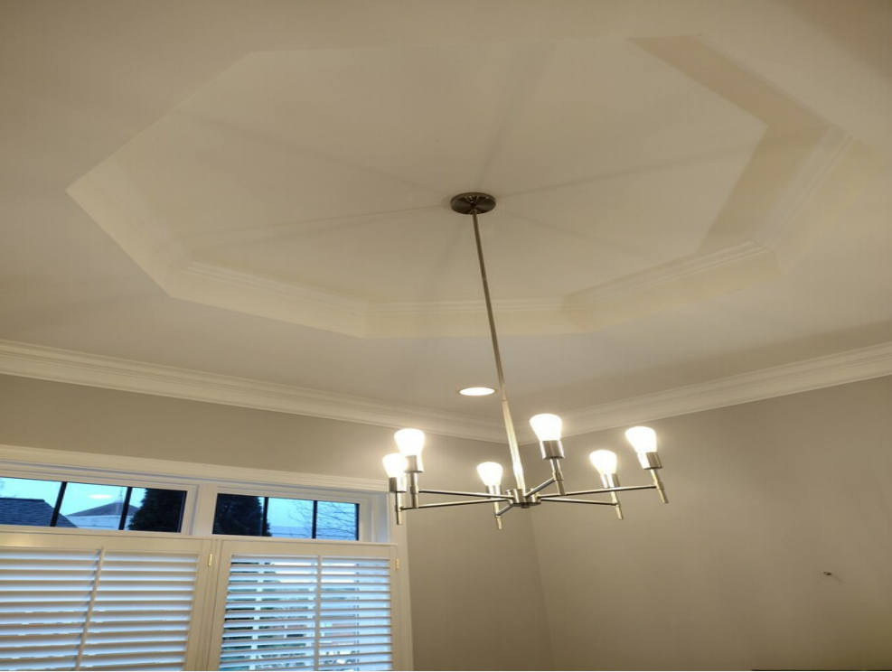
Ceiling - Reception Area
