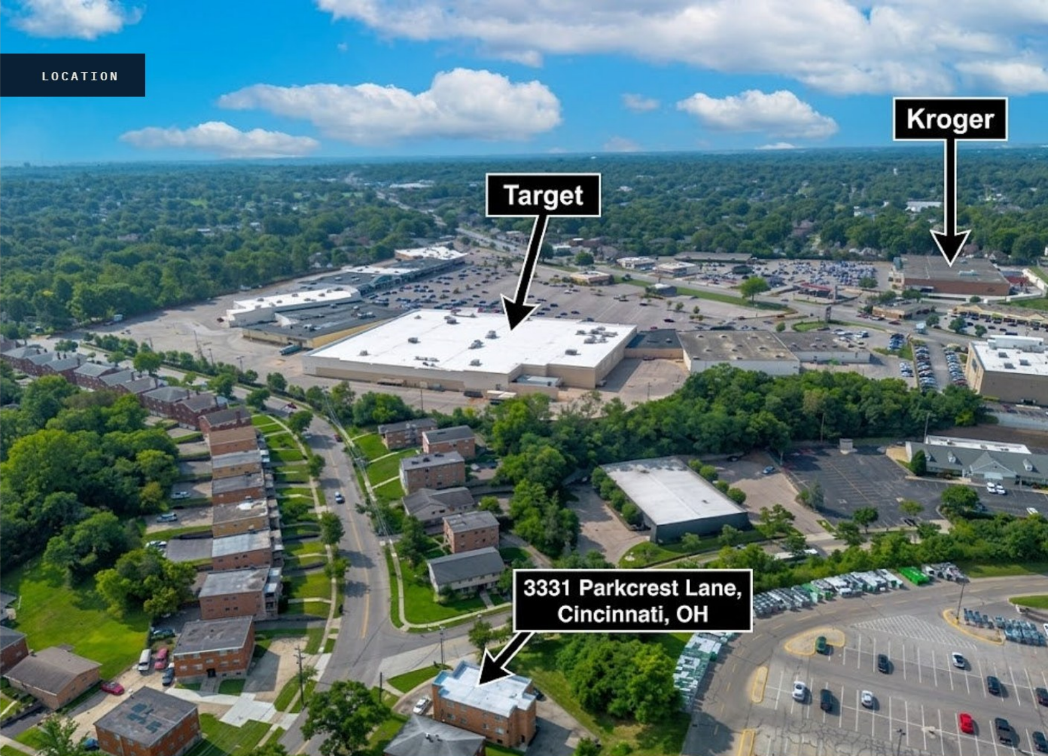
Parkcrest Lane sits behind the Glenway Avenue retail spine: Kroger, Target, Home Depot, and Planet Fitness all within walking distance of the building
