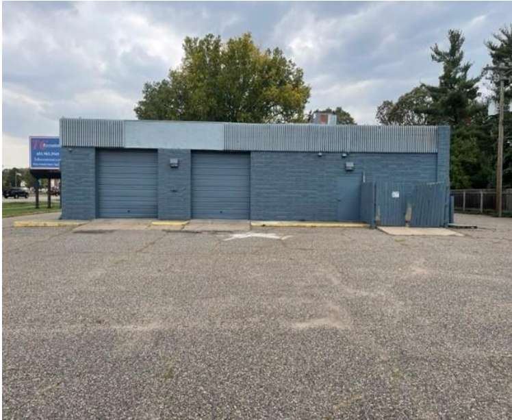
2 – 10' drive in doors
