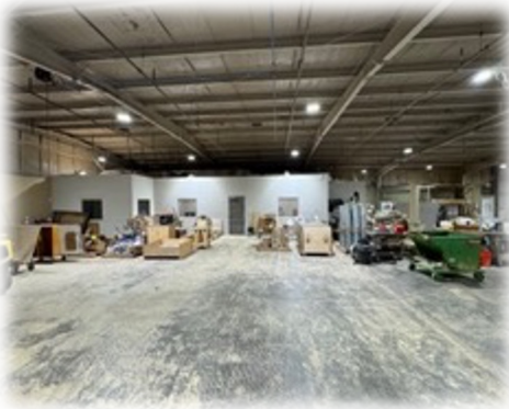
Sprinkler and fire alarm system
