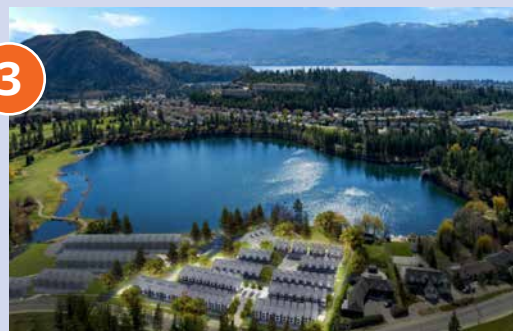
Project: Shannon Lynn on the Lake Townhouse community with 72 townhouses currently in the preconstruction phase.
