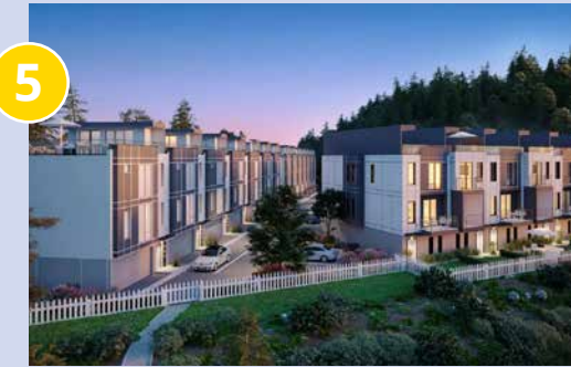
Project: The Arbor Townhouse community with 97 units currently under preconstruction.
