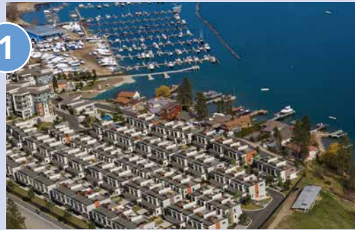
Project: Shelter Bay Townhouse community with 108 units currently under construction. Leasehold interest only.
